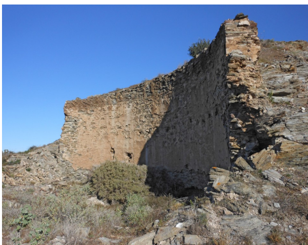
Carmen's baritel with the insets to support the beams of the whim.
