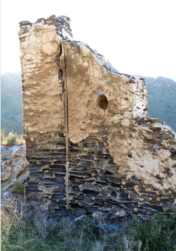
The beam seating in the masonry.
