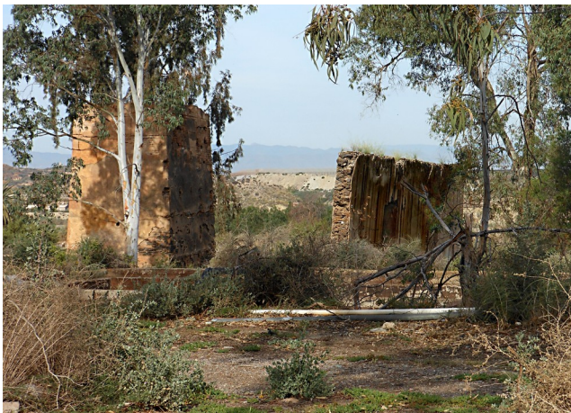
The boiler-house wall before demolition.
