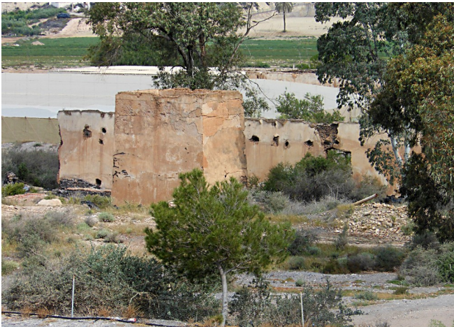
The extent of the boiler-house wall.
