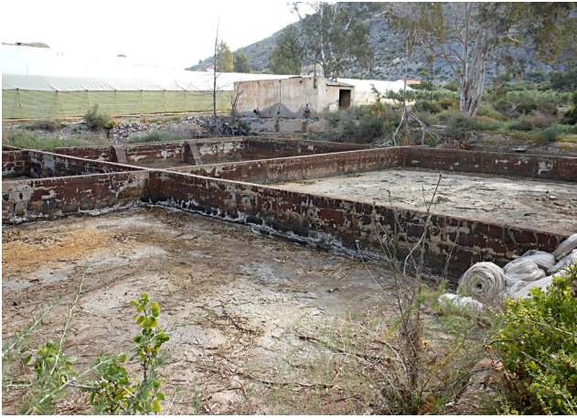
The tanks before their destruction.
