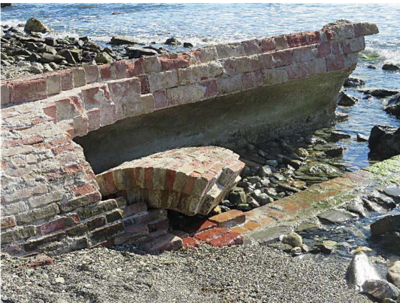
The rapidly deteriorating outfall pipe on the beach.
