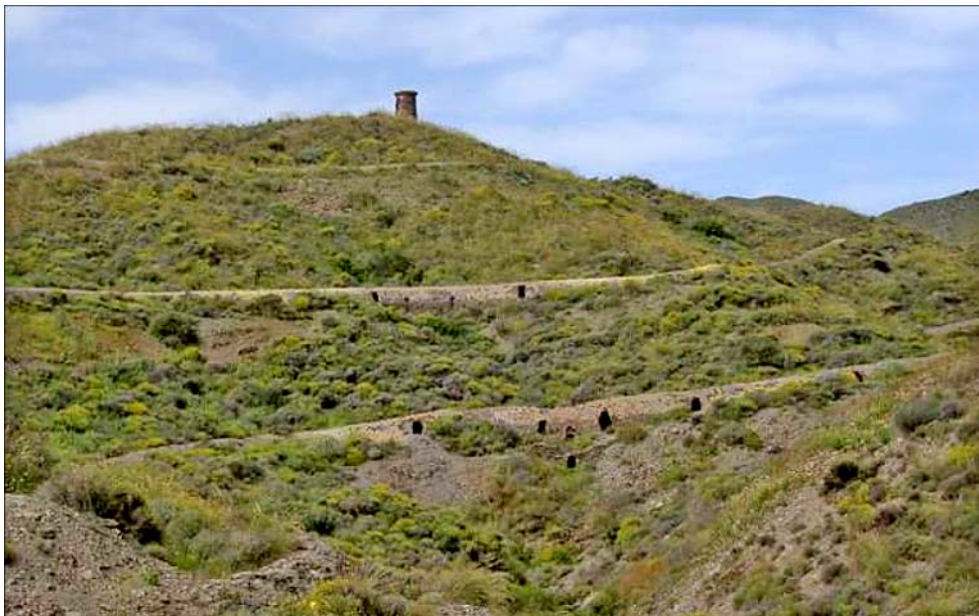
These condensation tunnels can be seen on the left shortly after passing the arches. Photo. mtiblog
