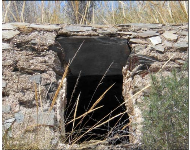
Inside the tunnel (left) and an entrance door (above).
