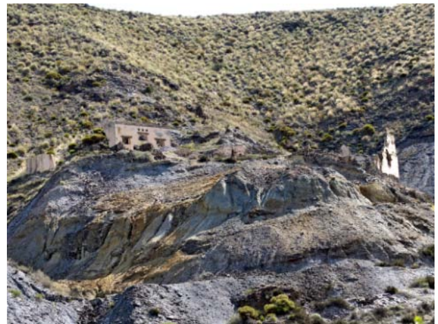
The transformer building.
