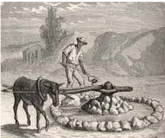
Simple mule-powered crusher.
