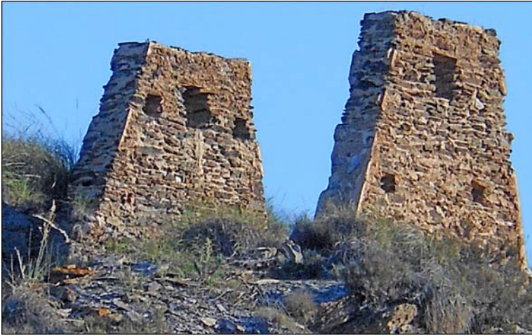
Aero cable supports on “Television Hill”.
