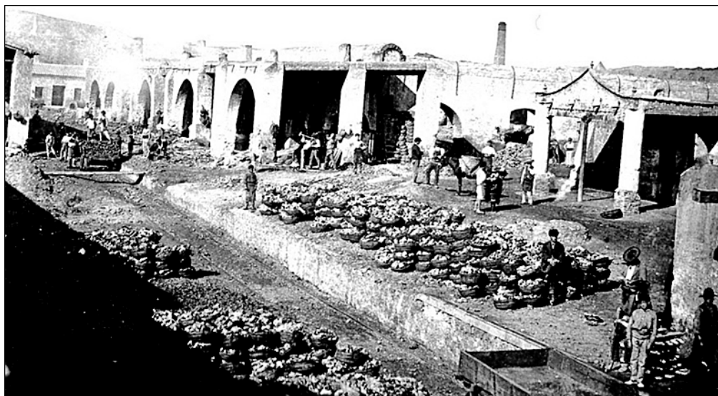
The esparto panniers can be seen in this photograph of the San Jacinto foundry at Las Marinas-Bolago near Pueblo Laguna.
