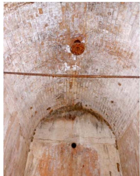
Inside the water tower.
