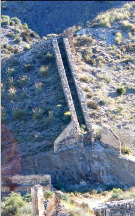
Left, the condensation channel from the boilers and, right, the ventilation channel running up towards Isabelita.
