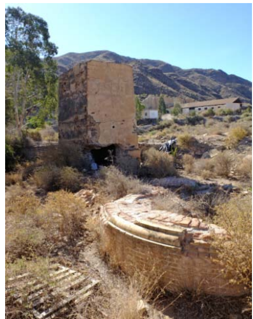
Right, the base of the chimney, in front of the water tower.
