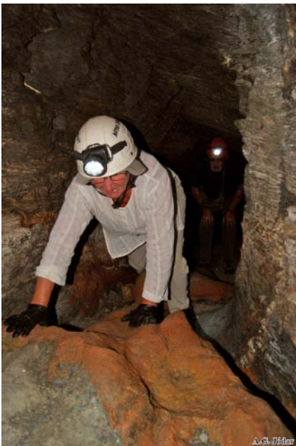
Left, the encrustations formed by the salts and minerals in the water can clearly be seen on the tunnel floor
