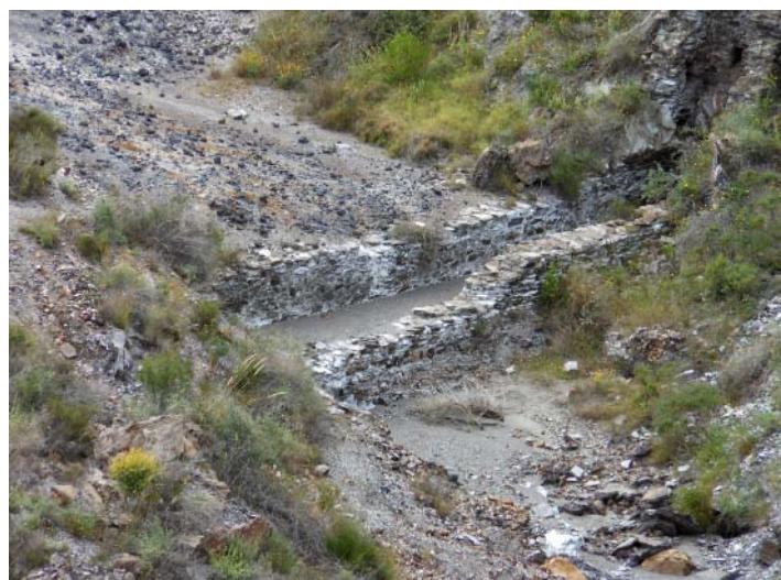
The entrance to the combined rain and pumped water tunnel is on the right.
