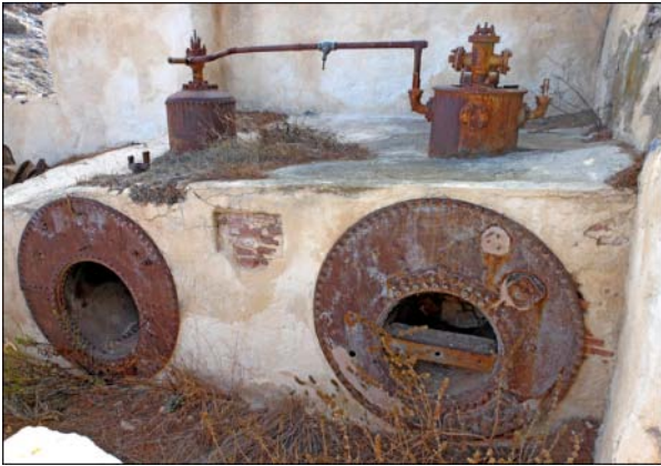
The small boilers favoured by Colson.
