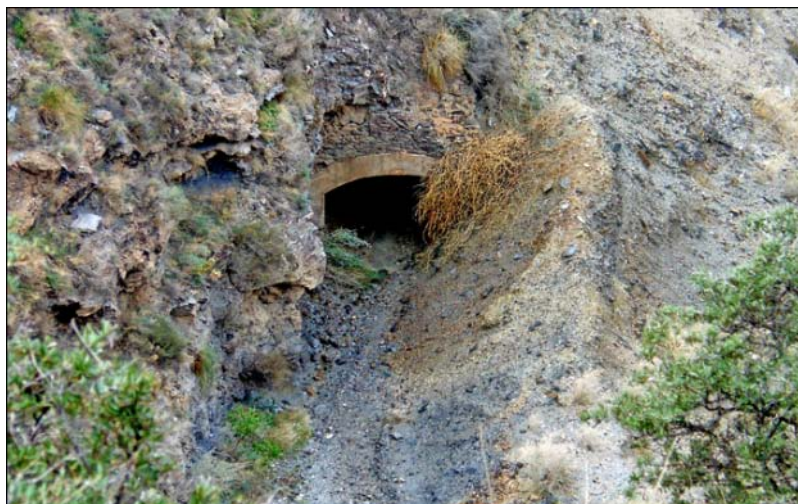
Archway at the end of the siding from the Santa Barbara tunnel that led into ...
