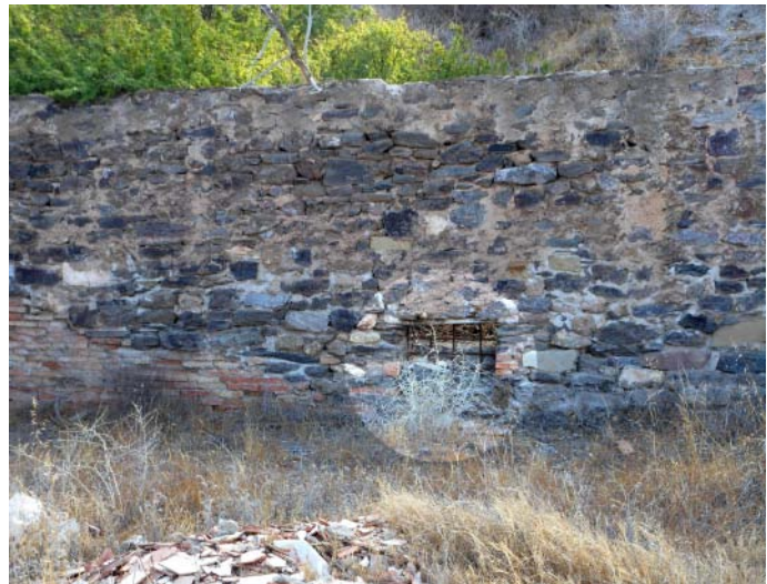
Above. The water left the courtyard through the grille (highlighted).
