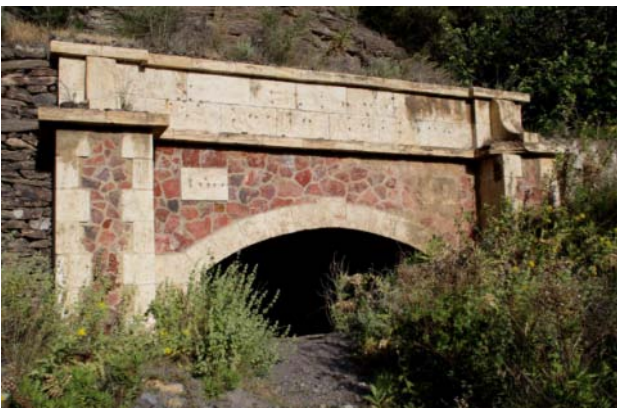
The entrance to the Santa Barbara tunnel.
