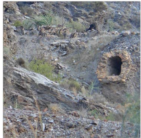
The water was pumped out through here.
