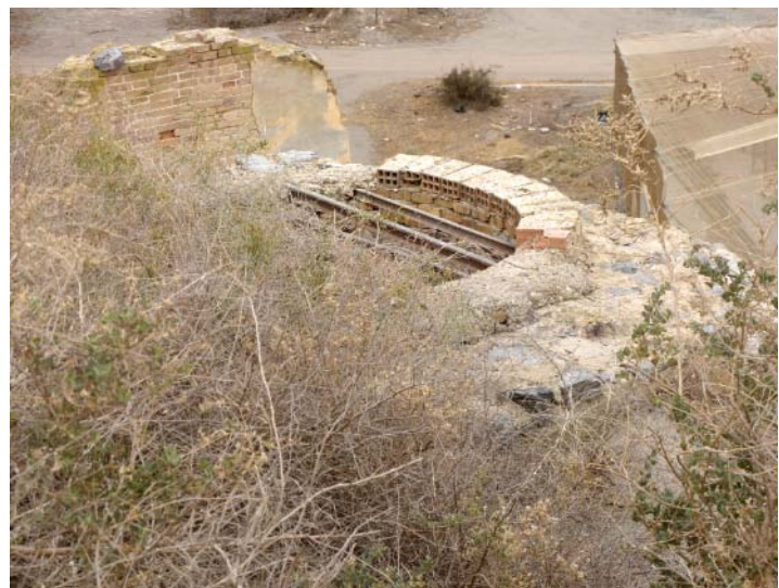
Left, back wall of Pozo Juala. This shaft has been remodelled many times over the years and is now completely sealed. Above, The top of the delivery shaft up which the water was piped to the surface.
