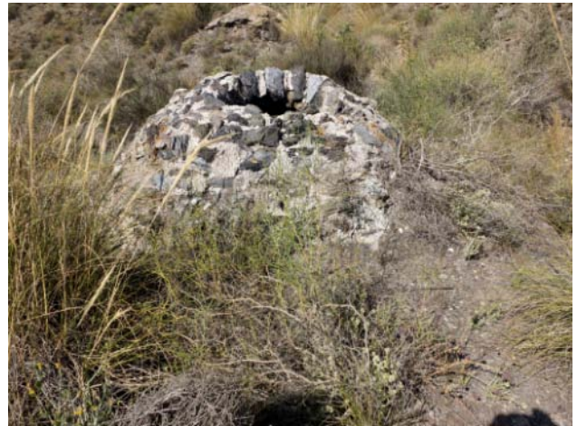
Ventilation shafts originally had domed caps. This is the only intact example I have found, hence the warning.
