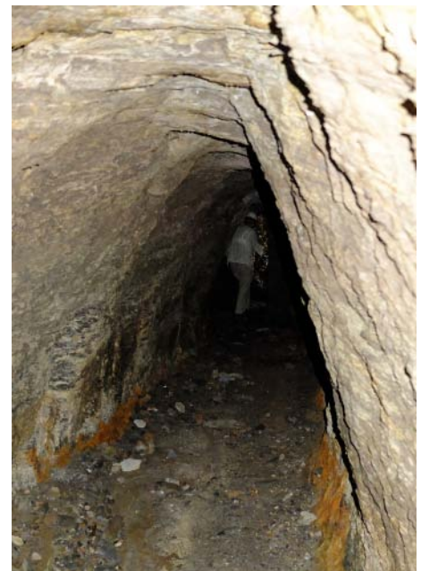
Left, the encrustations formed by the salts and minerals in the water can clearly be seen on the tunnel floor
