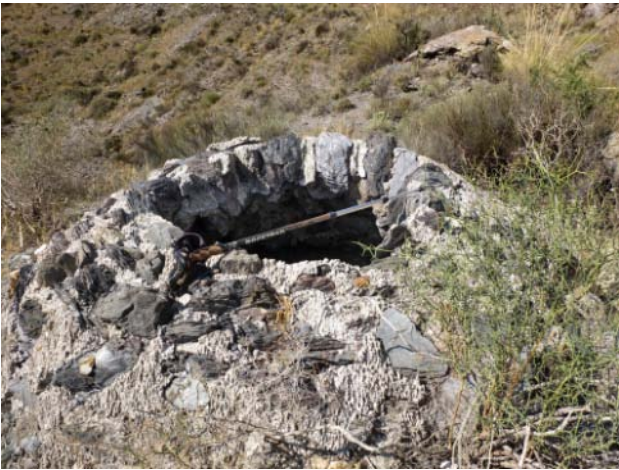
Ventilation shafts originally had domed caps. This is the only intact example I have found, hence the warning.
