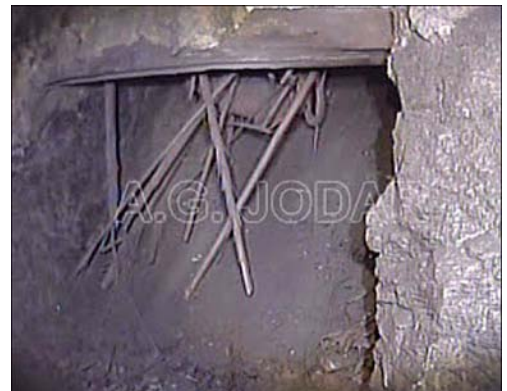
The ventilation shaft at the bottom of the main shaft. A fire could have been set in its base.
