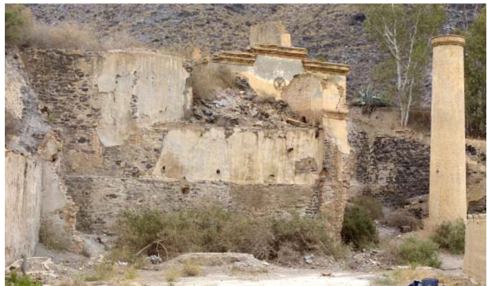
Above, all four shafts. The boiler room is on the left, the delivery shaft is above left, the remaining wall of Juala is in the centre with Encarnación above it and Ana on the right.
