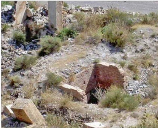
The San Juan shaft and the remains of the engine room
