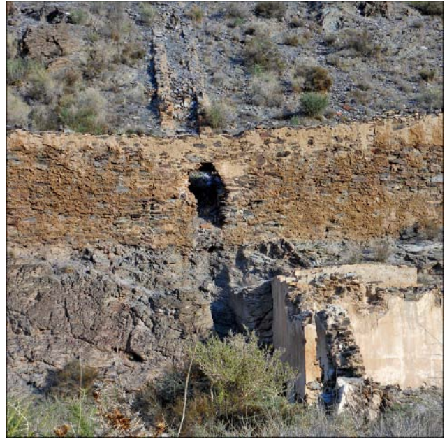
Left, the condensation channel from the boilers and, right, the ventilation channel running up towards Isabelita.
