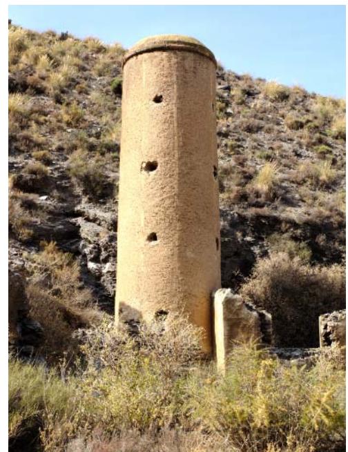
Right, the ventilation shaft. The chimney was added C1903.
