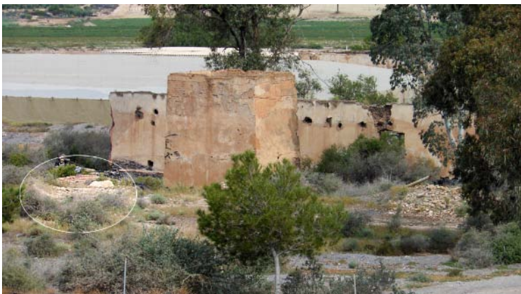
Above, general view of the power plant. The base of the chimney on the left is highlighted and the boiler room wall is behind the water tower.
