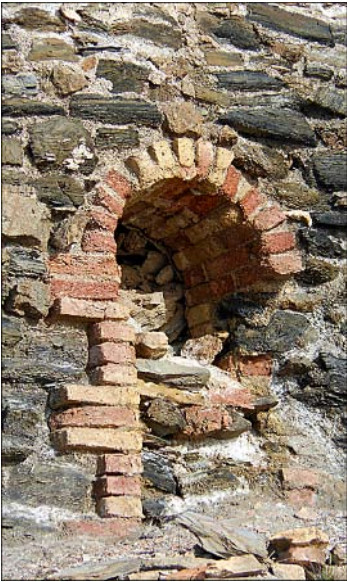
The other type furnace opening.
