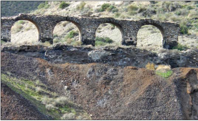
Remains of the arches of the Invincible foundry. All that is left of the furnaces can be seen at the base of the arches.
