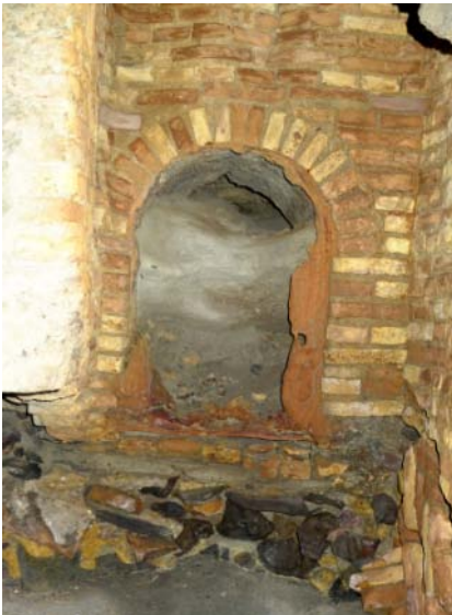
Left, water was probably pumped out through the lower aperture into the tunnel under the present course of the Jaroso rambla.
