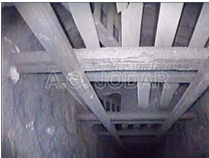
The shaft of the Independiente was used for access and extraction. The ladders and platforms can be seen behind the guide rails of the lift cage.
