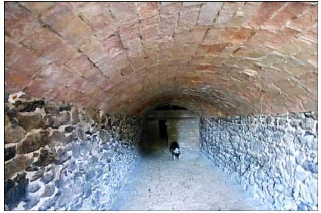
Start of the tunnel leading to the site of the compressors.
