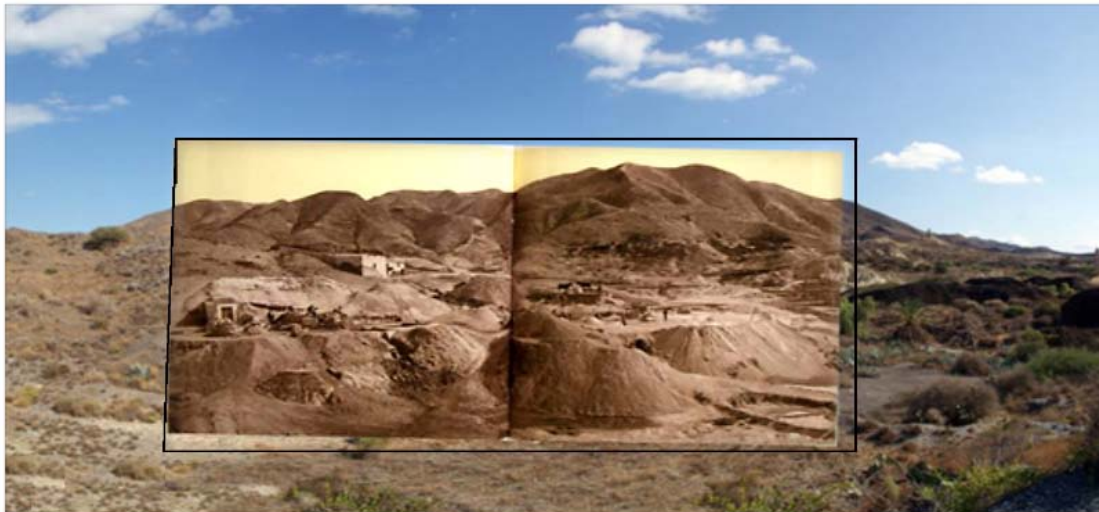
The washing plant, or lavadero, at El Tomillar. Photo montage A G Jódar using the original shown below by José Rodrigo.
