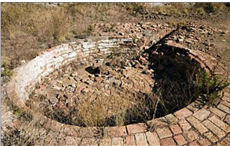
Detail of a rumbo showing the feed line.
