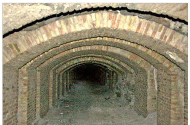
Just inside the tunnel. mti blog.
