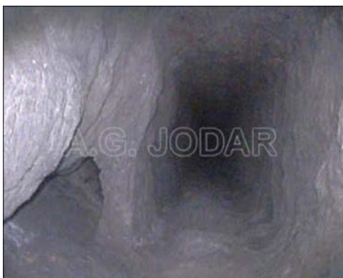
The ventilation shaft (on the left) in Elisa is separate. This is looking down from the top of the shaft.
