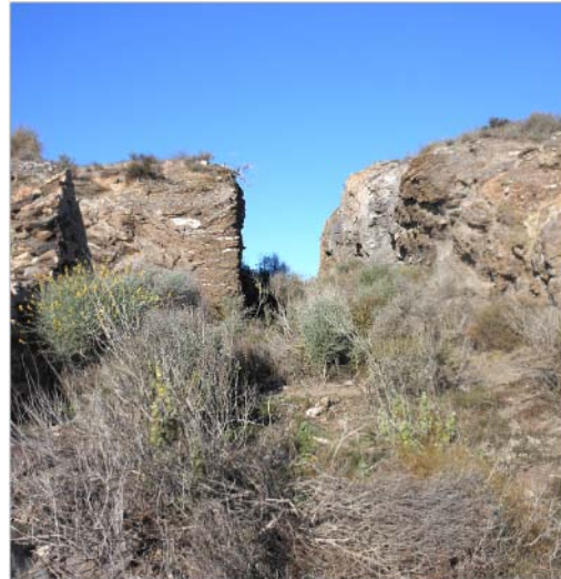
The cutting made for the buckets to clear the summit
