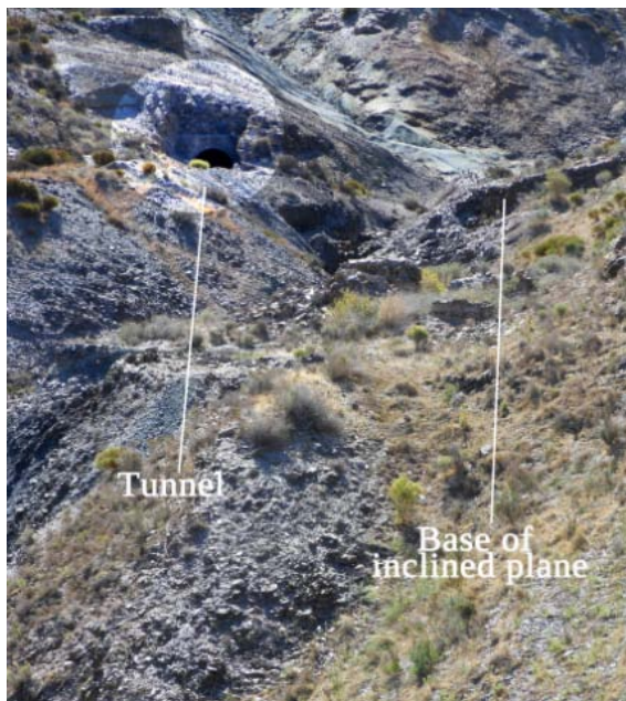
San Agustín tunnel. The base of the reversed inclined plane is on the right of the picture.
