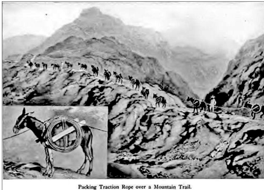
Packing Traction Rope over a Mountain Trail.
