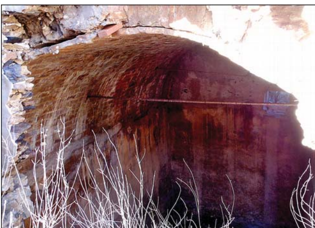
The roof of the aljibe is brick-lined and, possibly, constructed of stone.
