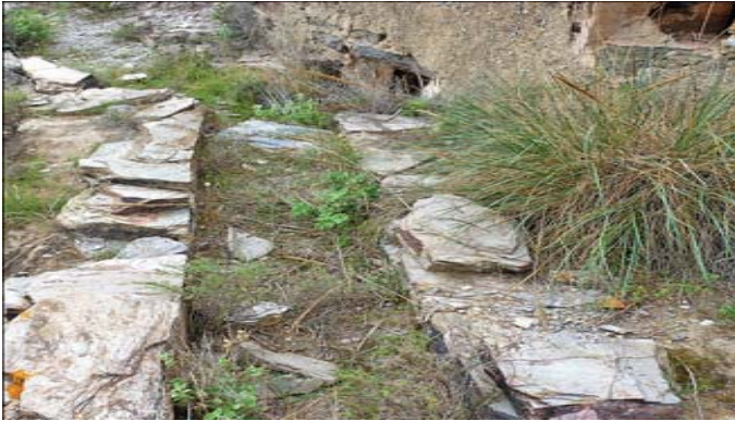
The roof run-off channel enters directly into the cistern.
