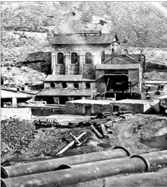
The desagüe in 1875. The original pumping engine was housed in the building to the front-right of the tall, later to be, engine house.
