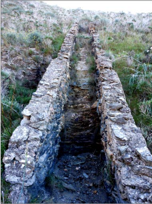
One of the channels used to collect water on the hillside. These used to be covered.
