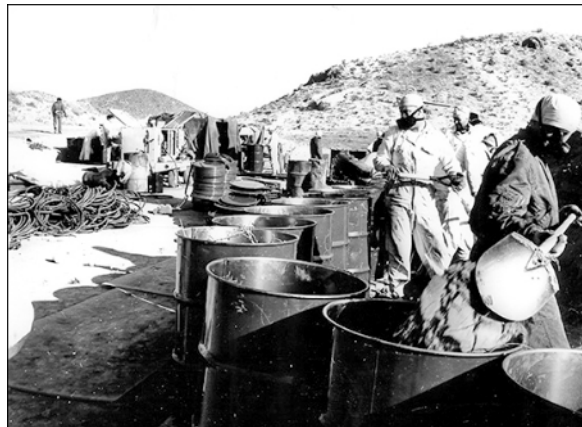
Shovelling contaminated soil into barrels for shipment to the U.S. Sandia National Laboratories
