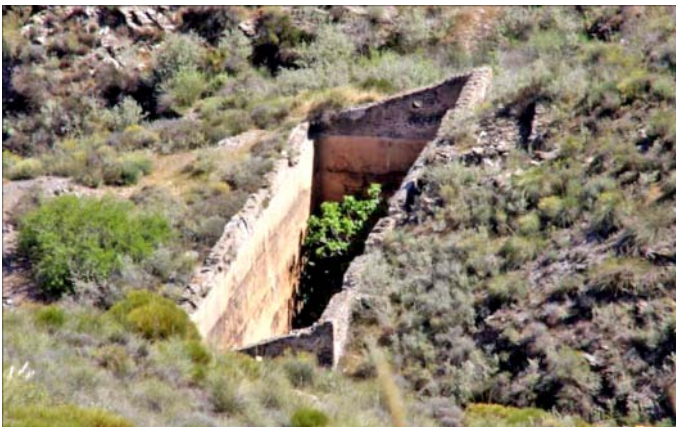
Two views of the Guzman balsa. To give some indication of size, I estimate its depth today to be about 7m. This is after a century of silt and rock being washed into it.
