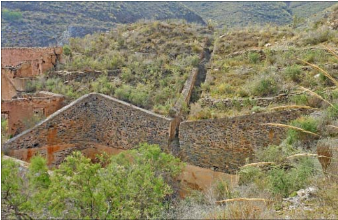
Two views of the Independiente's balsa showing the terracing and the feeder channel.
