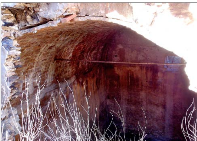
The roof of the aljibe is brick-lined and, possibly, constructed of stone.
