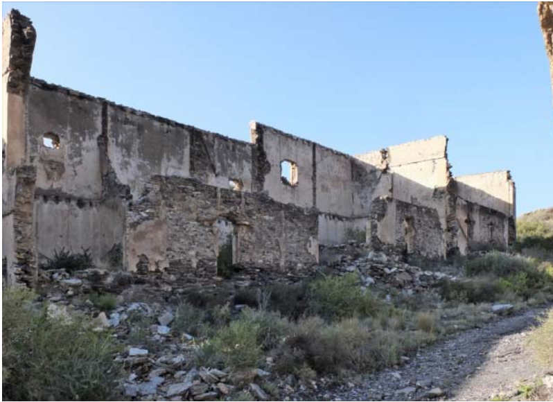
All that remains of the canteen and living quarters.
