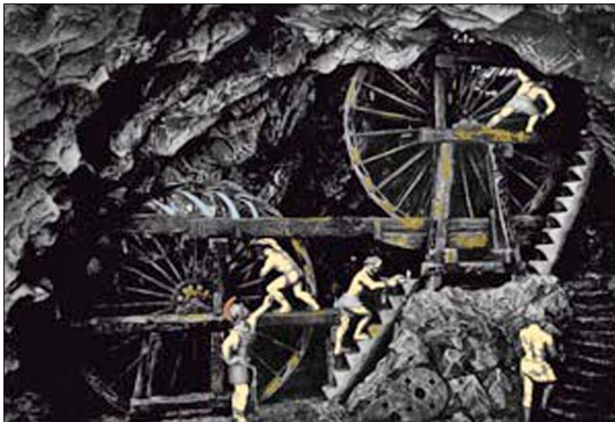
Slaves operating a water extraction system in a mine.
