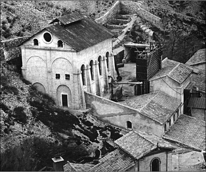
The pumping station in the Jaroso. Failure of the pumps saw the men frequently laid off with no pay.
