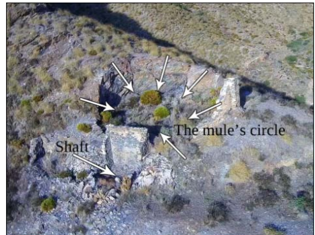
The mule walked round the central circle and the shaft mouth was behind the wall. Drone shot, A G Jódar
