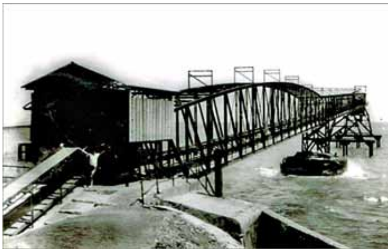
The conveyor entering the transfer tower, as can be seen there is no circuit and there is insufficient room to turn a truck. el abluelo facebook page
