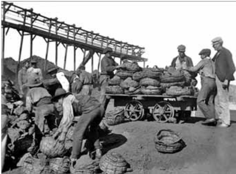
The Compañía de Águilas used loading piers and hand pushed wagons. The structure on the left is the extension of the aero cable terminal under construction.
