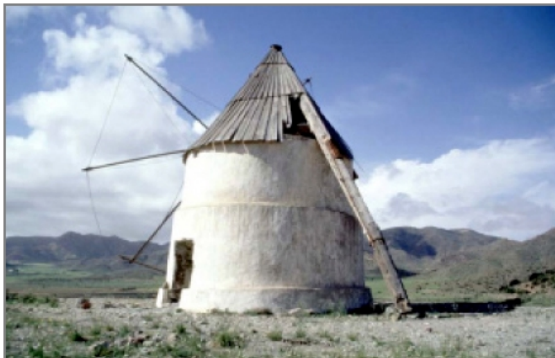
The guia can clearly be seen in this picture of the molino del Collado de los Genoveses with the ring of anchor pillars.
