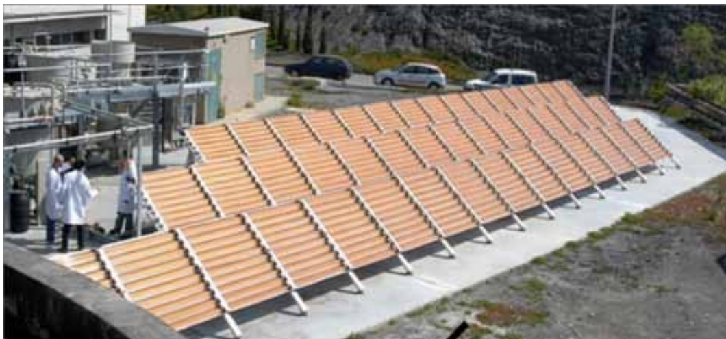
The photo-reactors at the depuration plant.
