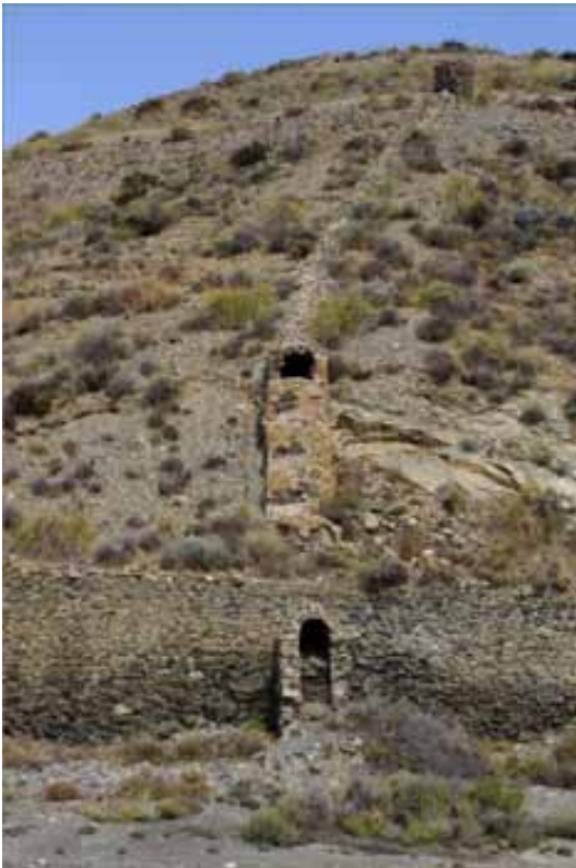
The stepped flue from the now disappeared calcination ovens.
