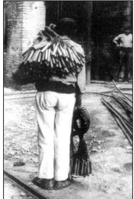
*The menchero carried the fuse cartridges to the barrenos.*
